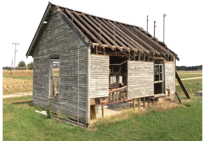
Figure 8. Shed in renovation process. Taylor M.
